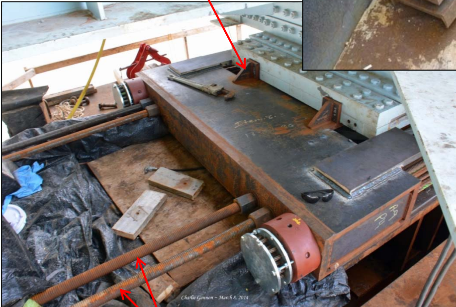
Pulling Rods to Trailing Bearing
